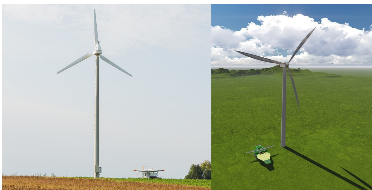
Figure 3: Conventional wind turbines next to docked AWE systems of comparable rated power: photo of the TwingTec pilot system [35] (left) and rendering of the envisioned offshore system of Ampyx Power, the AP4, with a rated power of 2 MW [36] (right).
